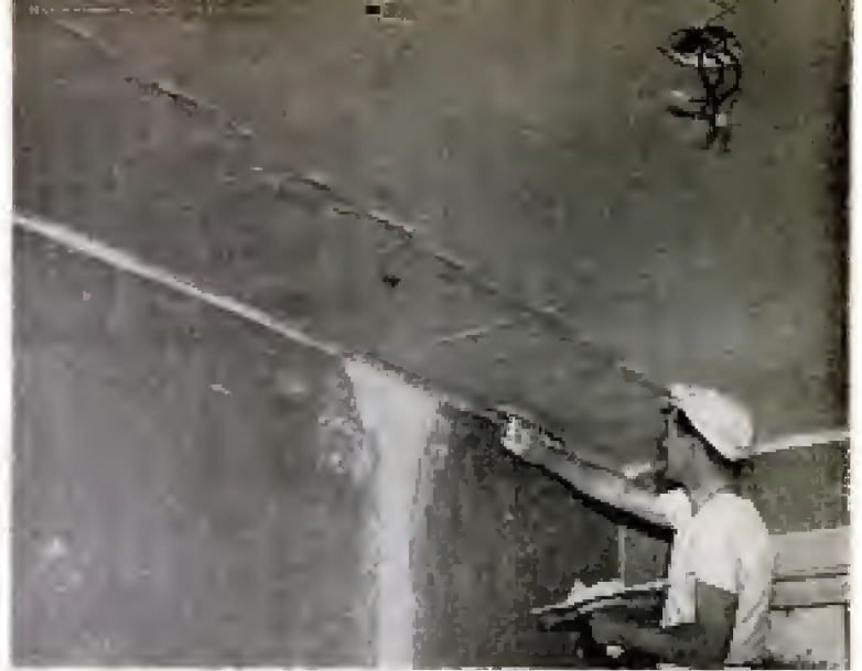
Last of base coat is being troweled on ceiling. Note above how plaster is troweled toward center of room. Light weight of ready-mixed plaster makes job easy
